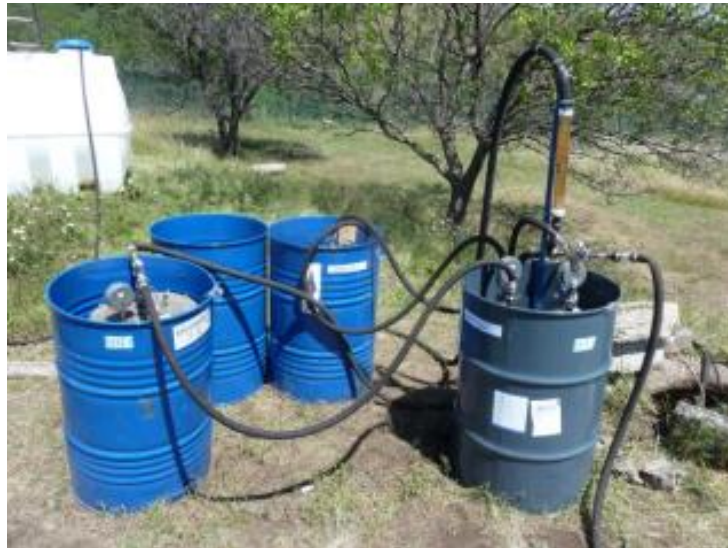
Fig.2 The water purification at Saakadze site
