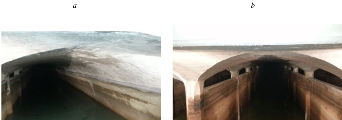
Figure 3. Internal view of first - a (1911-1917) and second -b (1928-1932) reservoir structure.
